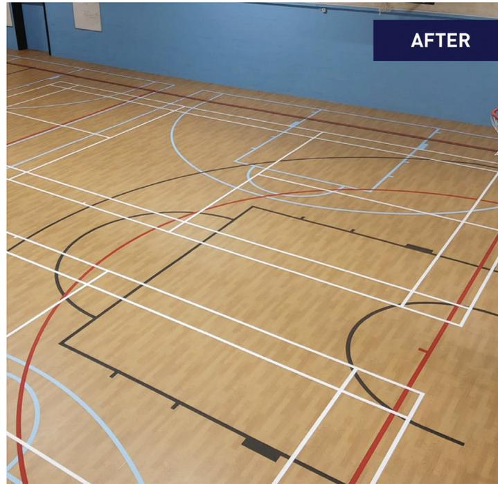
"The Isolsport underlay also supplied by Gerflor, enabled us to lay the Taraflex® Multi-Use directly over the existing concrete floor, this was a real benefit as the project was on a very tight schedule, due to the hall being required for exams."
