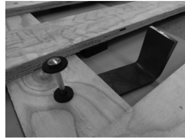
Hammer the pin into place.
