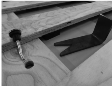
Place this wedge beneath the sleeper before hammering the anchor pin.
